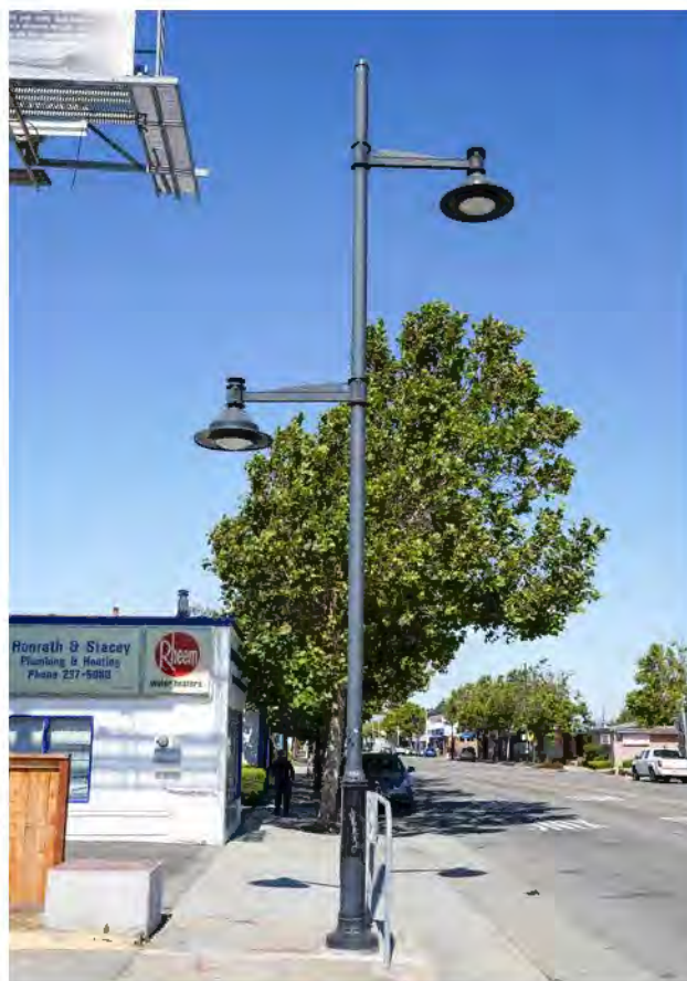
Street Lighting featuring dedicated illumination for both the roadway and the sidewalk
